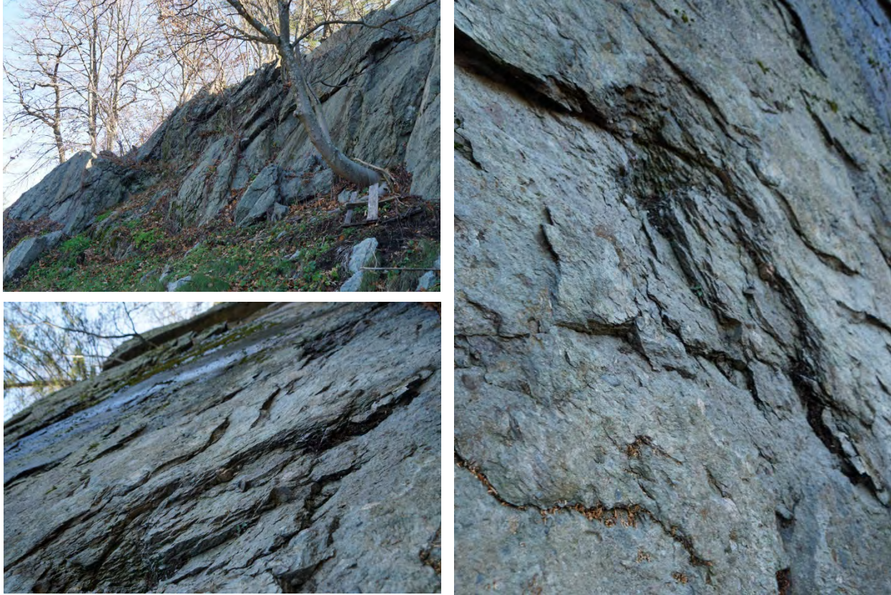
Different views of the cleavage in the quarry face. Angle of the cleavage is about 75^\circ and strikes roughly east-west.
